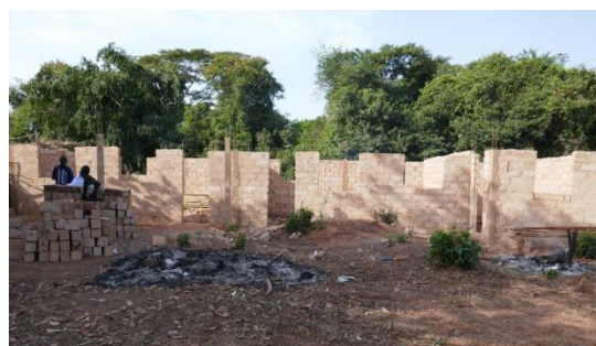
School in aanbouw in Gantamba
